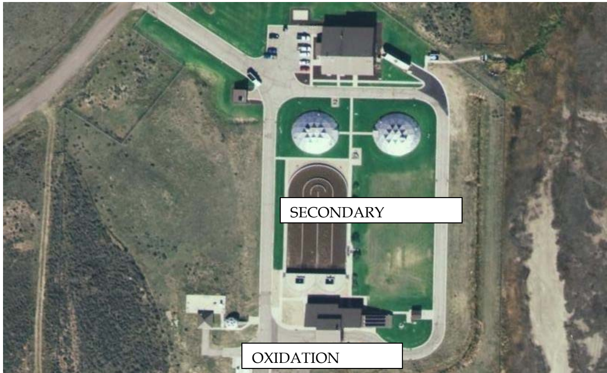
FIGURE 2 Aerial View of the Facility (Source: Google Earth)
